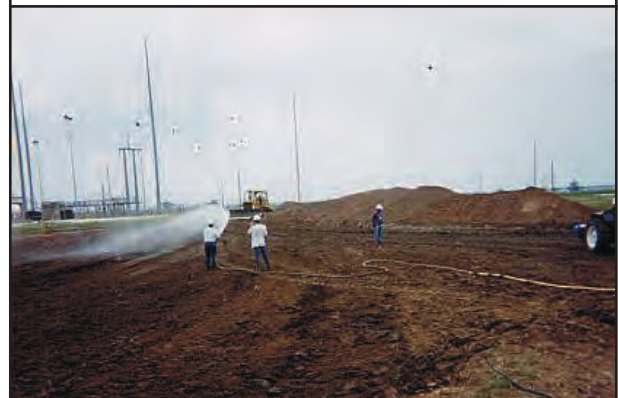
Department of Energy, July 15, 1999. Following application of Bio-Matrix bioremediation systems ppm hydrocarbons dropped to 573.
